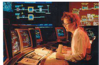
Remote management solutions including SCADA, networking, Telemetry and Industrial Modems.
