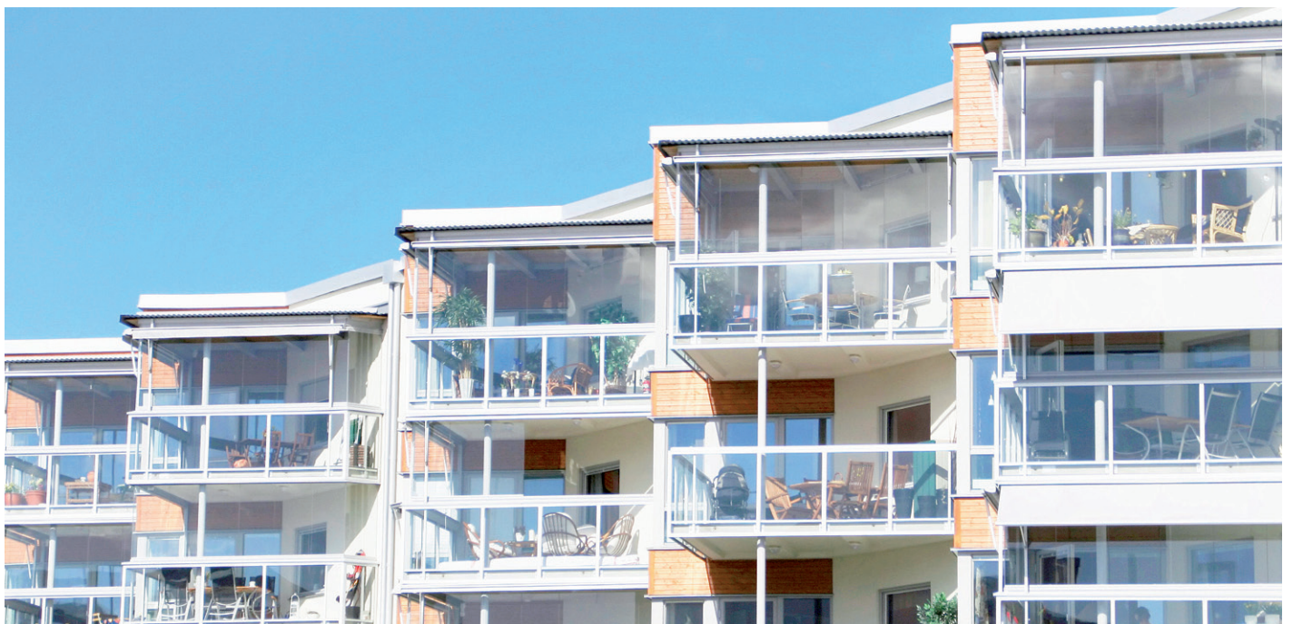
Landlord sub-metering offers clear cost-saving opportunities for the tenants, at the same time as it benefits the environment.
